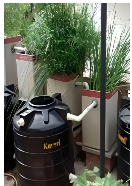
Grey water treatment setup at houses, to manage water judiciously
